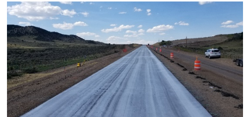
SH 13 & CR 6 – Reconstruction
