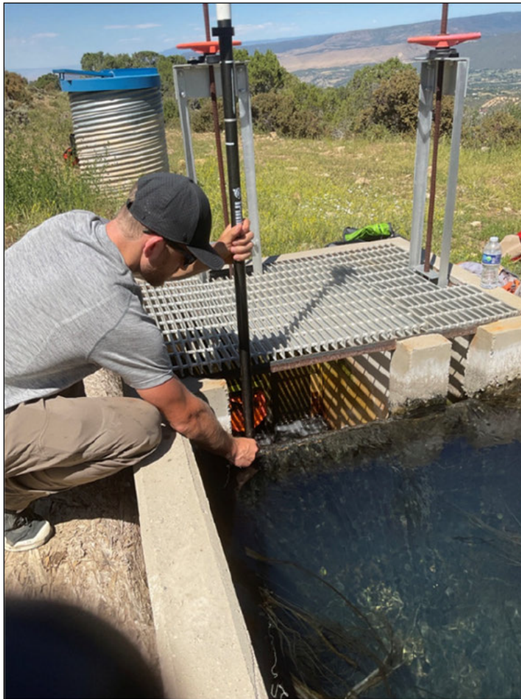
Figure 13. Photograph of German Creek Splitter Box.
