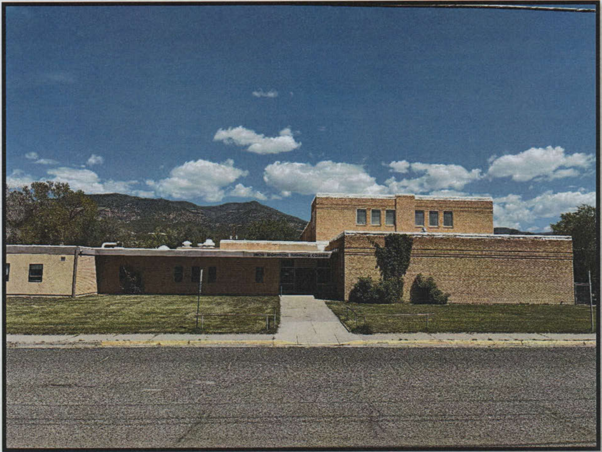
Looking north from 4 th Street.
