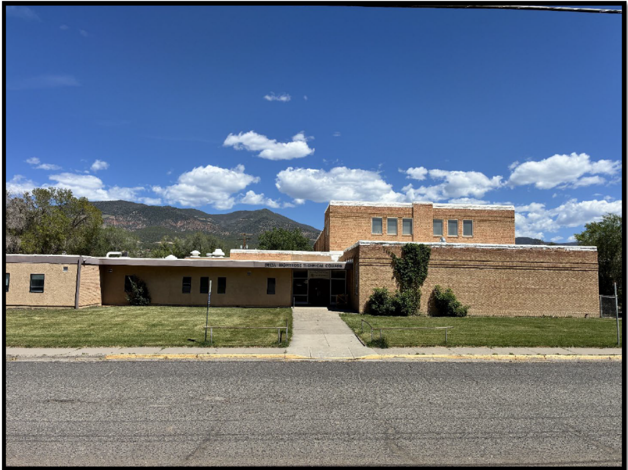
Looking north from 4 th Street.
