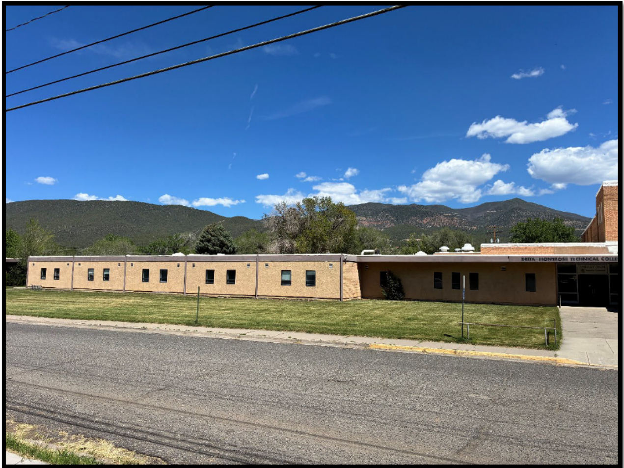
Looking north from 4 th Street
