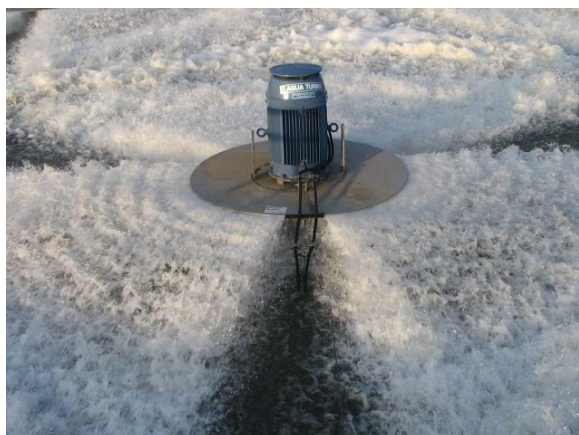
Discharge is directed away from the motor.
