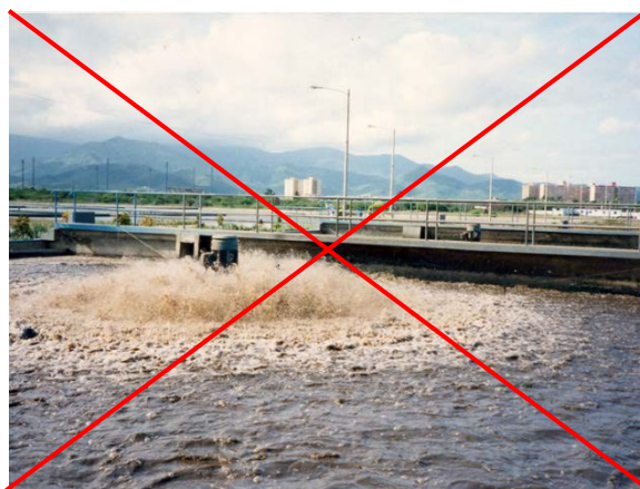
Excessive spray, aerosol, odor, and vapor draft.
