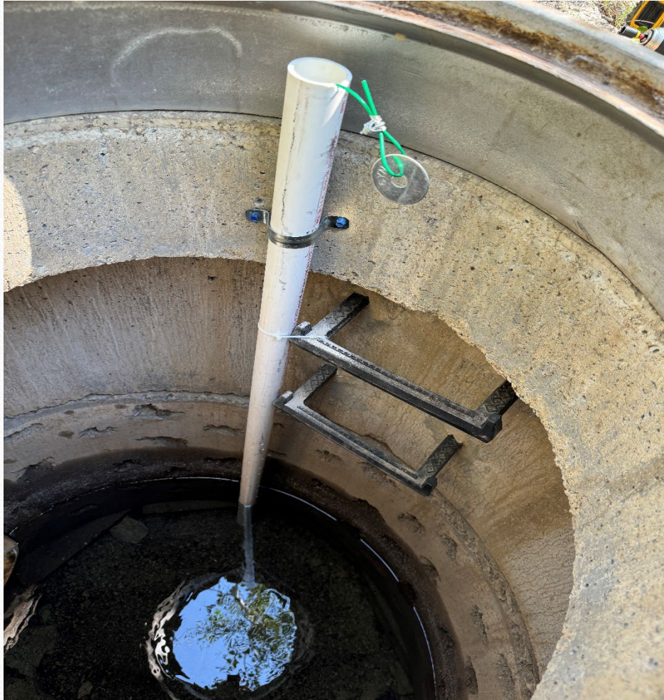
Installation of pressure transducer at Lake Fork Spring Box
