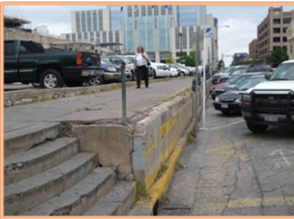
Before: Image of sidewalk and steps.
